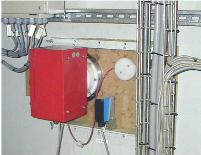
Illustration 5: measuring moisture in the fibre silo
